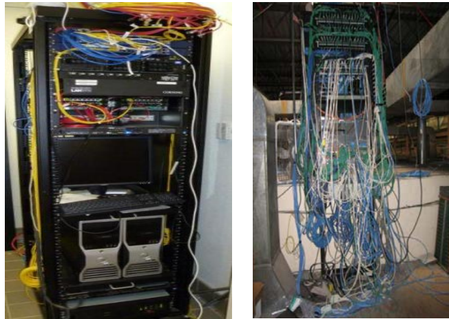
Figure 2. Poor Industrial Network Installation Can Generate Unacceptable Downtime Risks
